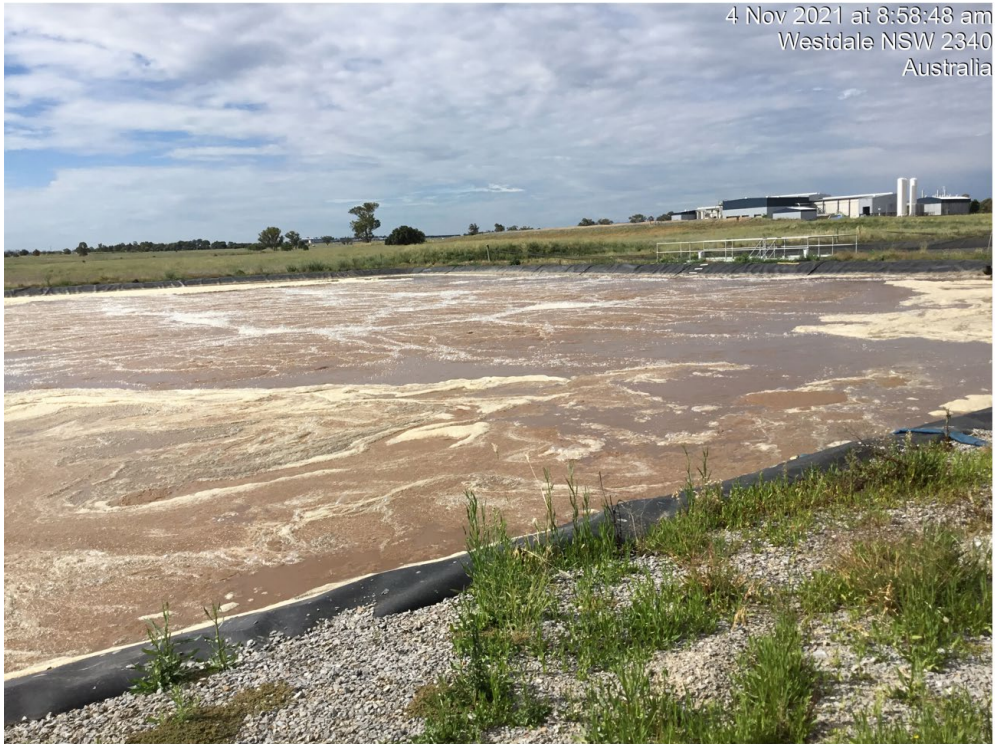
Photo 3: View looking southeast over wastewater pond towards the main plant
