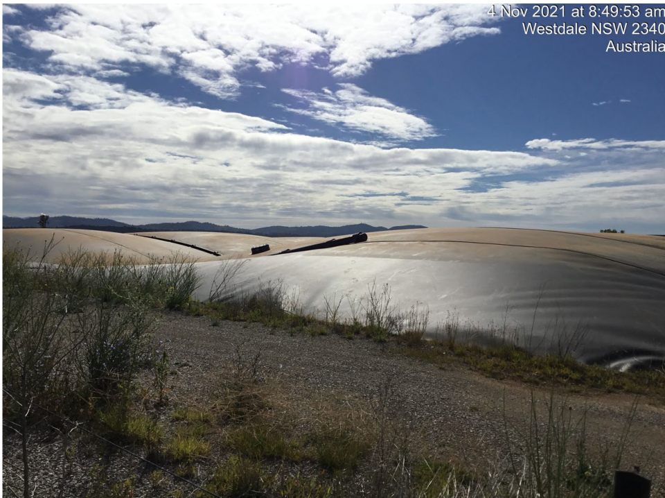
Photo 6: View looking east across some of the covered anaerobic lagoons (CAL)
