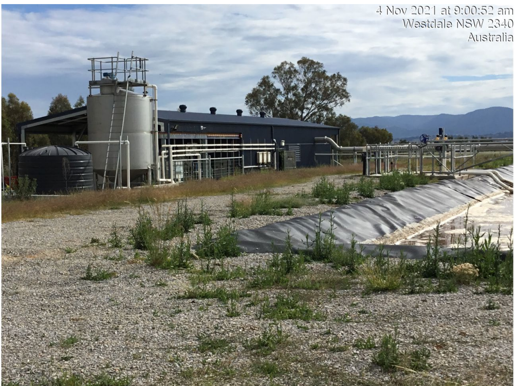
Photo 2: View looking northwest towards the wastewater treatment plant
