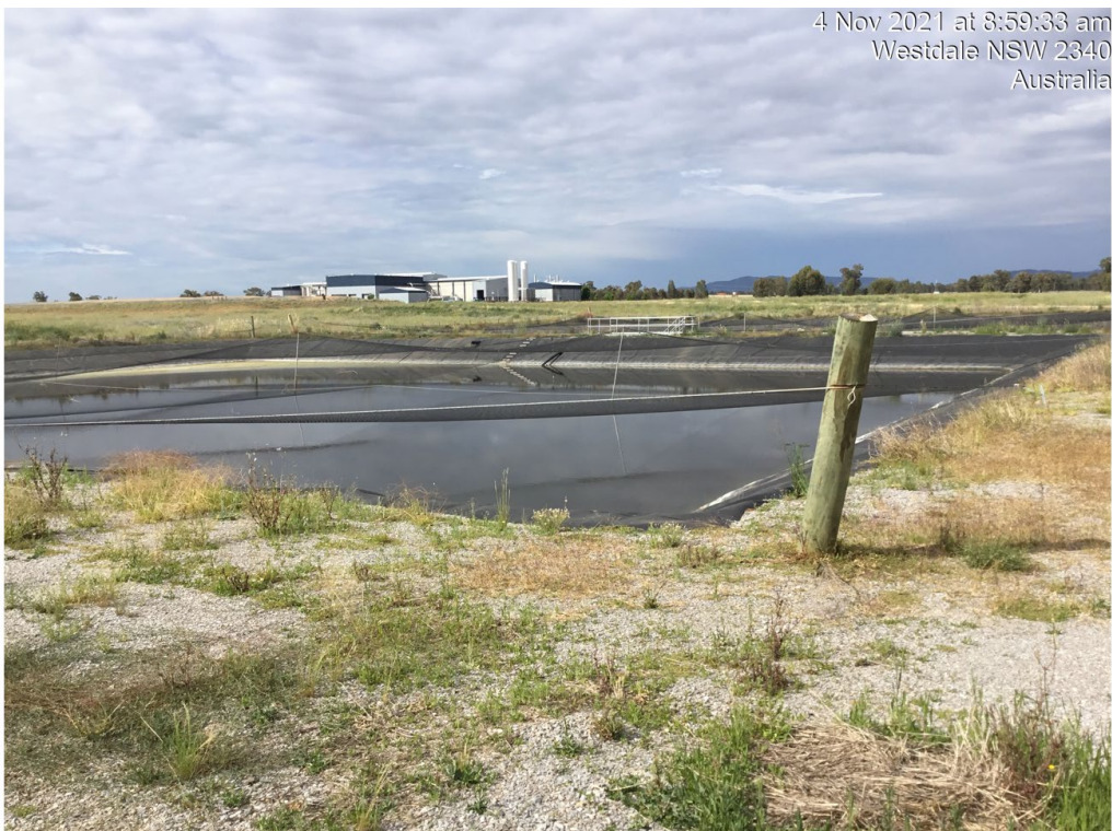
Photo 4: View across one of the wastewater ponds with bird netting
