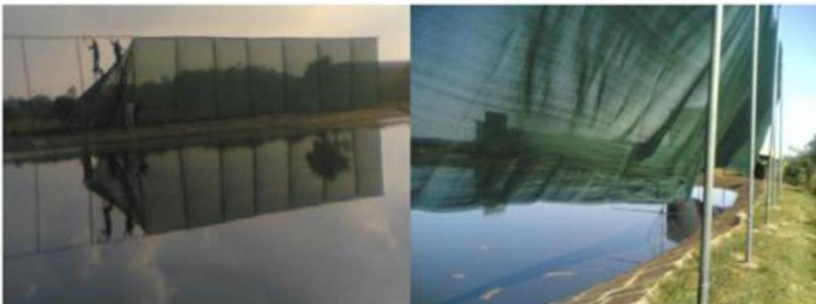
Figure 2 - Example Image of spray curtain design to mitigate overspray in accelerated evaporation
