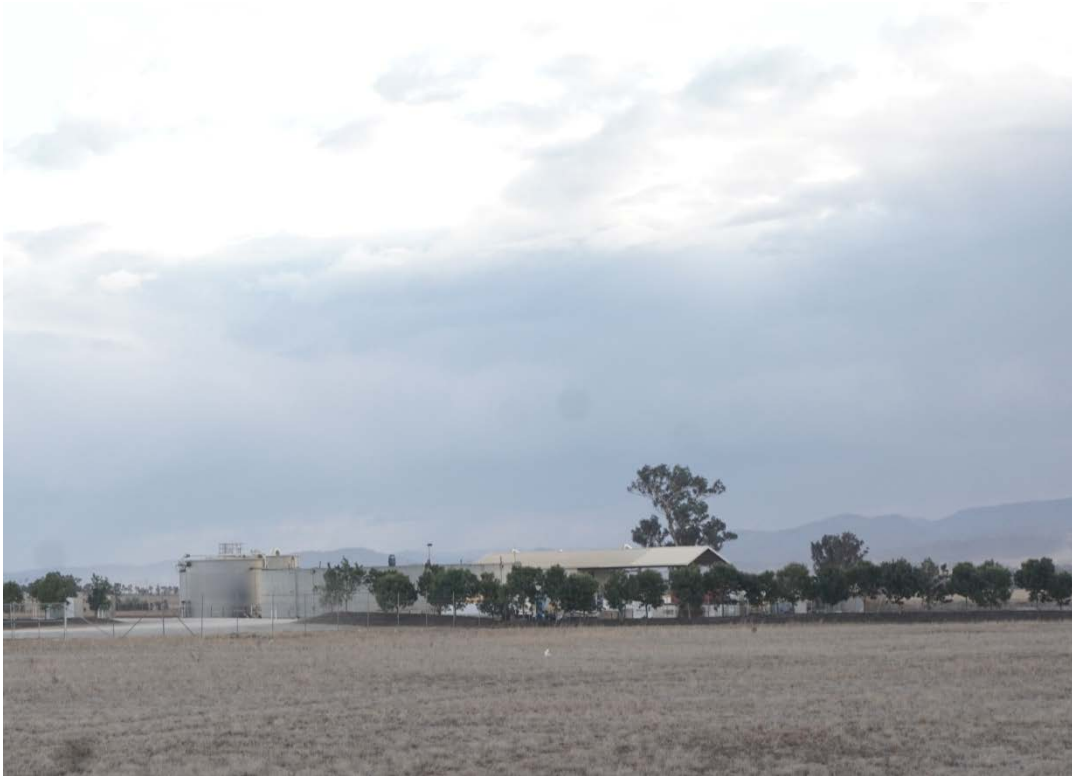
Photograph 3 Existing waste water treatment plant
